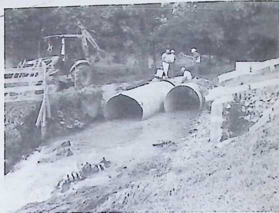
Flooding in Rockbridge County washed out roads and bridges. In this photo, VDOT officials work with a private contractor to make temporary repairs to a bridge near Walkers Creek.
